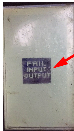
ELECTRIC CONNECTION ANOMALY IN PROGRESS
